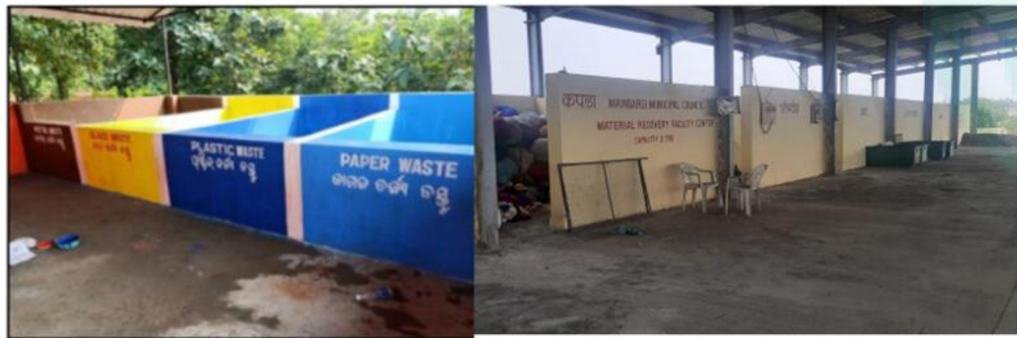
Storage compartments for dry waste
